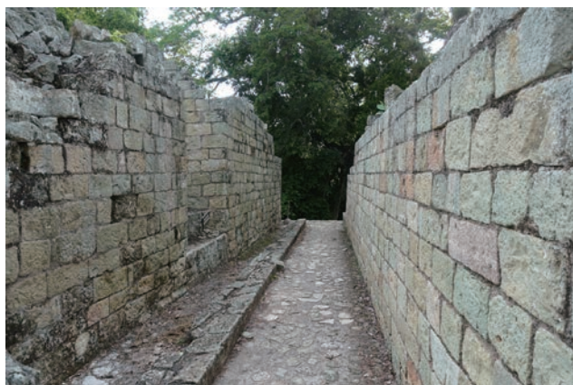
Figure 7 Structure of the upper passageway of Temple 11
