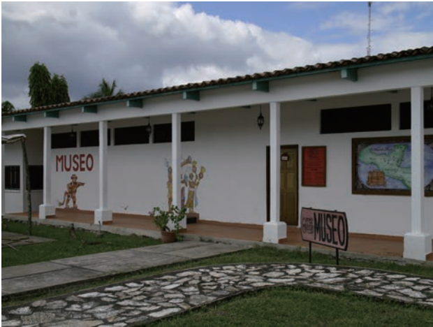
Fig. 3 Exterior view of Casa K'inich Children's Museum
